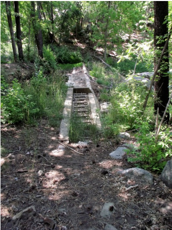
Diversion Dam in Groom Creek
